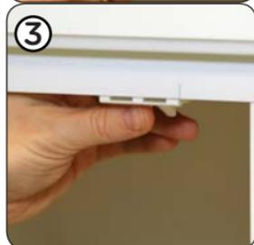
4. Hold the Mounting Plate VERTICALLY with the arrow pointing up and slide the Perfect Installation Tool into the top position by pushing on the Locking Tab.
