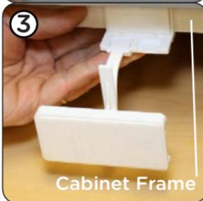
4. Push drawer in so you can judge to make sure the mounting plate doesn't hit on a screw head. Reposition, if needed.
