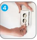
Choose the Standard or Decora Insert depending on your Wall Plate style, and fit Insert into the Mounting Plate
