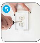
Place Mounting Plate and Insert over the outlet with the Qdos logo at the right side and secure firmly with provided screws.
