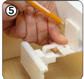
5. Carefully mark the location for the SureCatch™ on the frame with a pencil.
