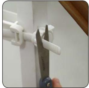
After cutting, use the Tightening Tool to loosen the Tightening Nut until the cut ends of the straps are protected behind the Tightening Nuts.
